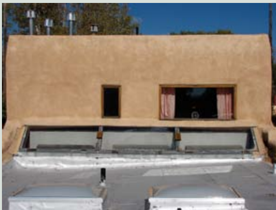
This rooftop clerestory isn't pretty, but you never see it. It captures the solar energy which heats the water tanks below to 100 degrees on a decent solar day. (see photo right).
