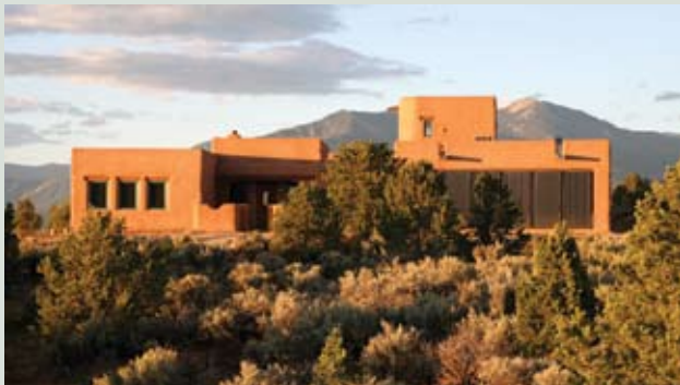
The collectors pocketed into the garage wall heat this entire 2,200 s.f. pumice-crete home
