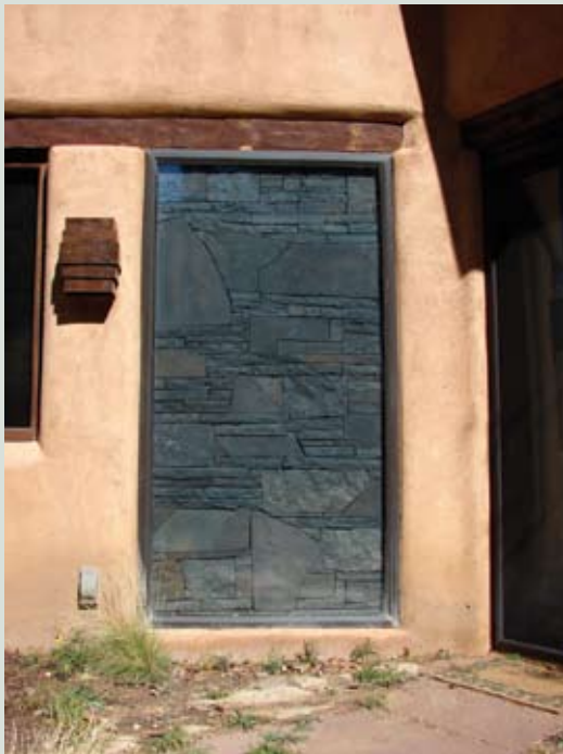
This trombe wall radiates heat into a bookshelf-lined study.
